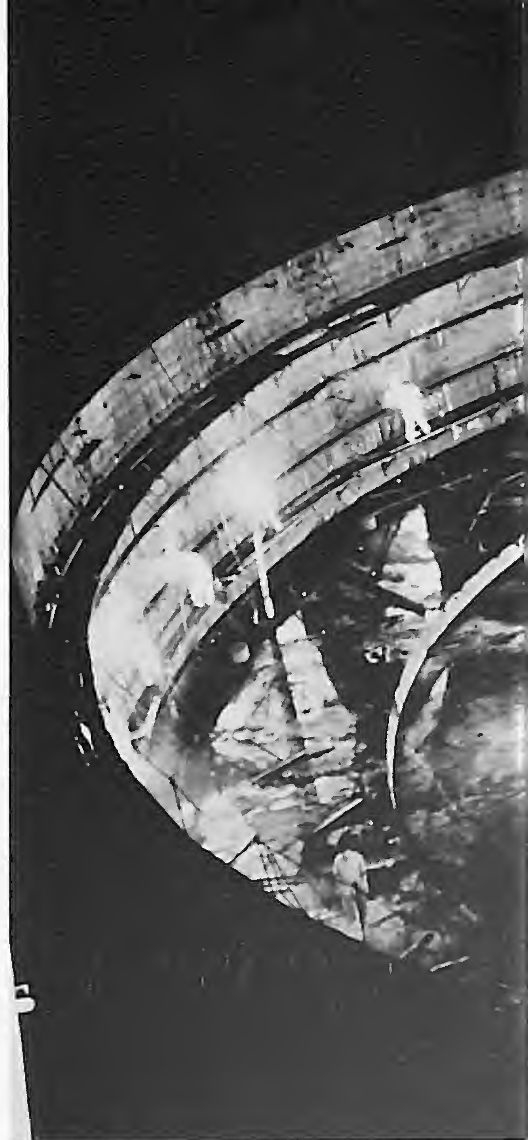
Welding a giant oil tank.
